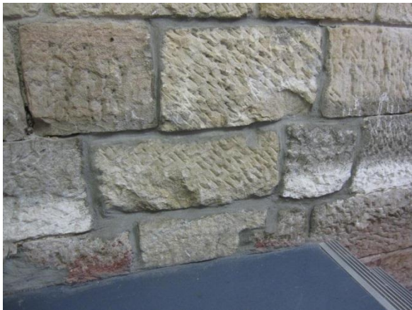
DETAIL OF CEMENT POINTING TO LEVEL 2 STONEWORK
