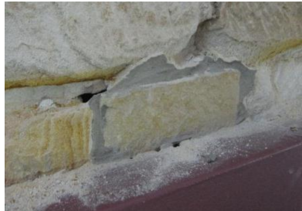
PATCH REPAIR WITH STONE VENEER ABOVE THE BUILT OUT BRICK WALL (LEVEL 1)
