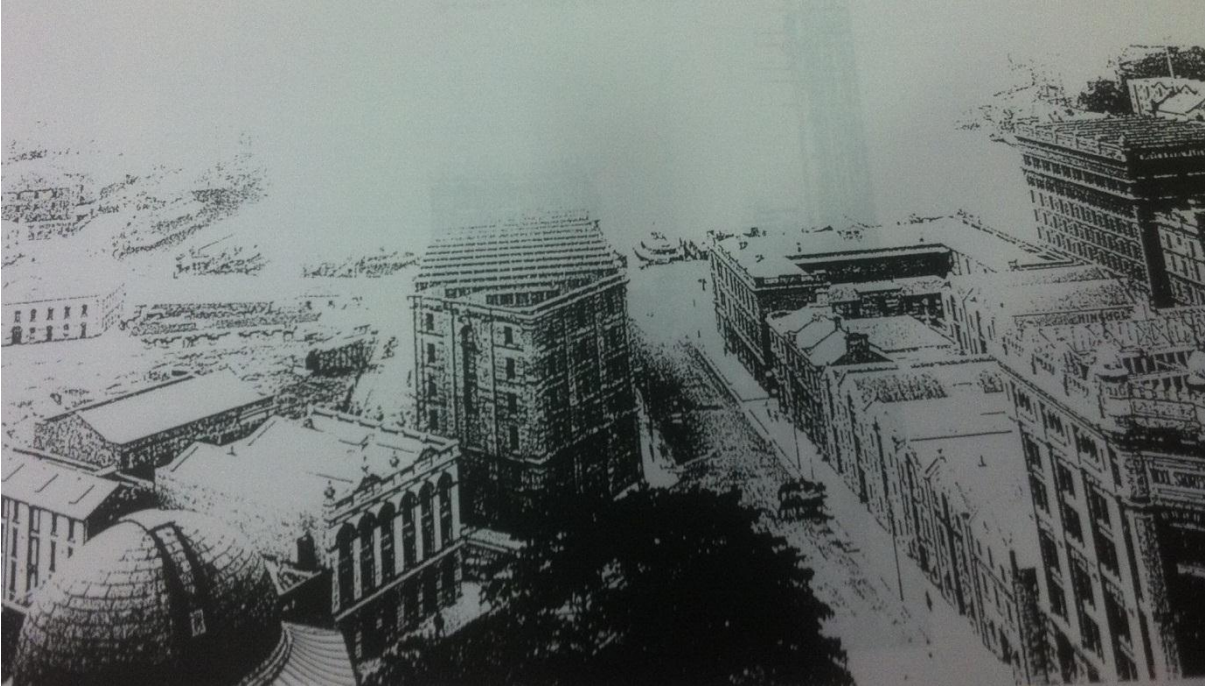
FIGURE 34 – VIEW OF THE F L BARKER WOOL STORES FROM THE LANDS DEPARTMENT BUILDING, 1890
