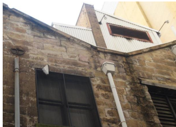
DETAIL OF STEPPED CRACKING SUGGESTING MOVEMENT ALONG THE ROOFLINE AND SPALLING TO PARAPET
