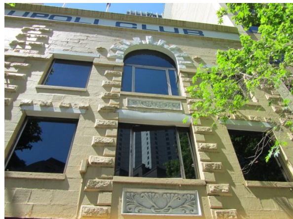
DETAIL OF THE FAÇADE OF NO. 14 SHOWING THE ALTERED WINDOWS AND C.1910 ART NOUVEAU SPANDRELS WITHIN THE INFILLED CENTRAL BAY
