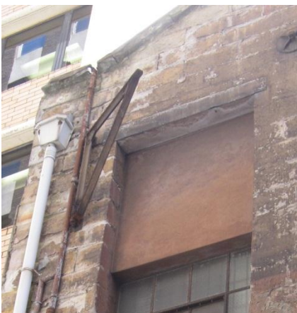
DETAIL OF THE REMNANT JIB HOIST AND INFILLED WINDOW (TO FIRE STAIR)
