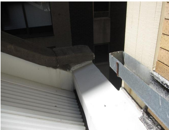
DETAIL OF BOX GUTTER, SOUTH WALL GUTTER AND DISCHARGE TO THE REAR LOFTUS LANE (SE CORNER)
