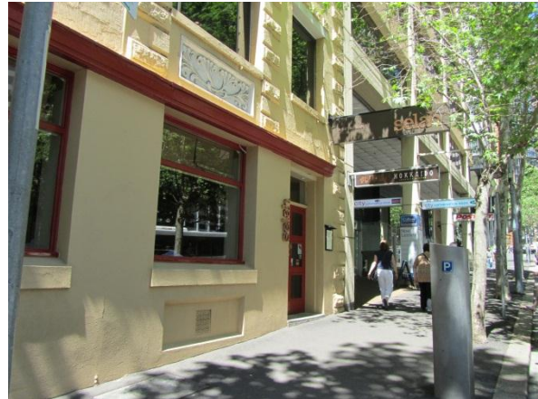
GROUND FLOOR SOUTHERN STORE (14 LOFTUS STREET) SHOWING THE C.1910 ENTRY AND REMNANT TIMBER WINDOW FRAMES. THE ORIGINAL QUIONS AROUND CENTRAL BAY HAVE BEEN REMOVED
